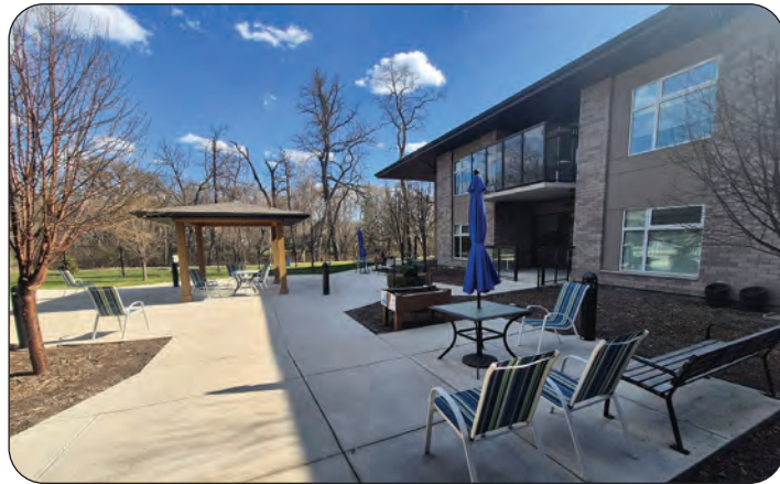
Completed phases of the Boyne Lodge have allowed the campus to expand to 103 personal care beds, two respite rooms and a growing range of seniors services as plans move ahead for a future assisted living facility.
