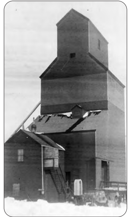
PHOTO SUBMITTED The Mollard elevator was a landmark for travelers along highway #3 for 34 years.
